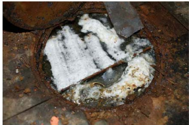
Photo 10. Photograph of heavy microbiological contamination in basement cell system in auxiliary vault. The degree of contamination in this area is so heavy that some air samples were overloaded.
