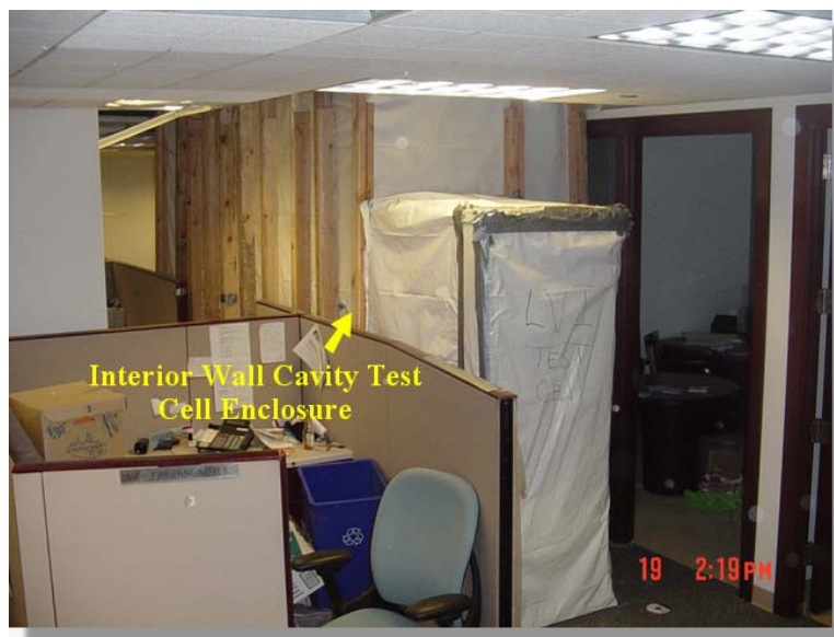
Figure 1. Example of an interior wall cavity cell
