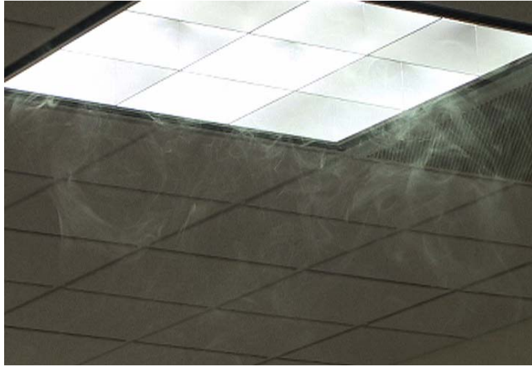
Figure 4. Interior cavity pathway.
