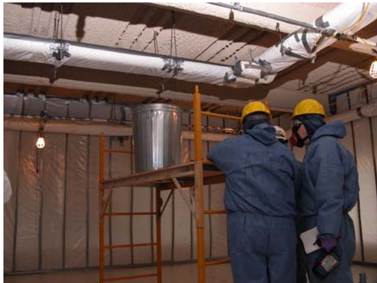
Figure 2. Preparation for the Cell System raceways smoke test.
