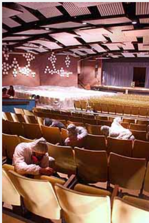
Erin Kiernan Workers steam clean seats in the auditorium. Later, cloth samples are removed to insure asbestos does not exist.
