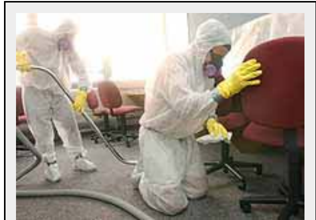
The News-Times/Wendy Carlson Asbestos removal cleaners vacuum up and wipe down equipment in the computer room at Brookfield High School.
